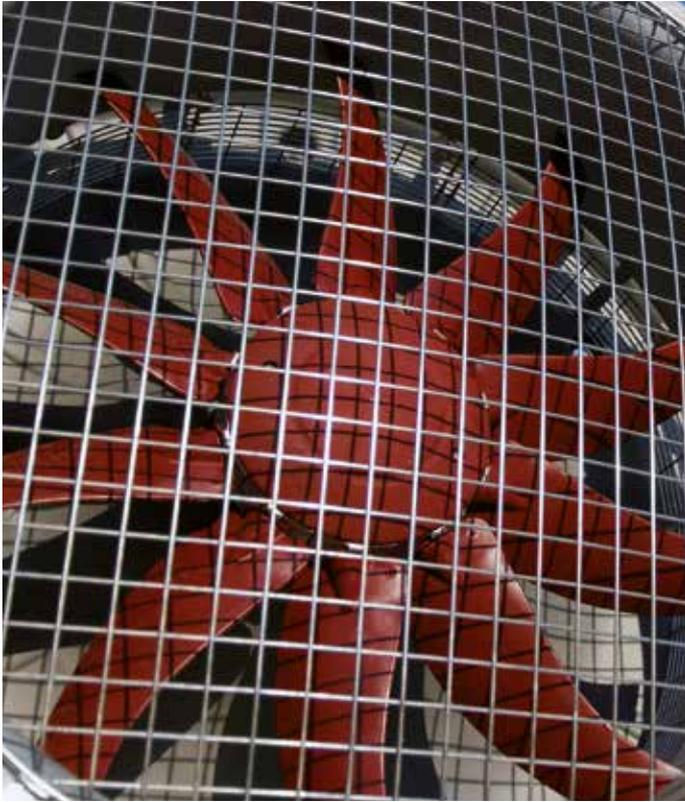
The main function is that of extracting air from closed environments by means of centrifugal or axial fans and conveying this air outside via ventilation ducts and chimneys.
