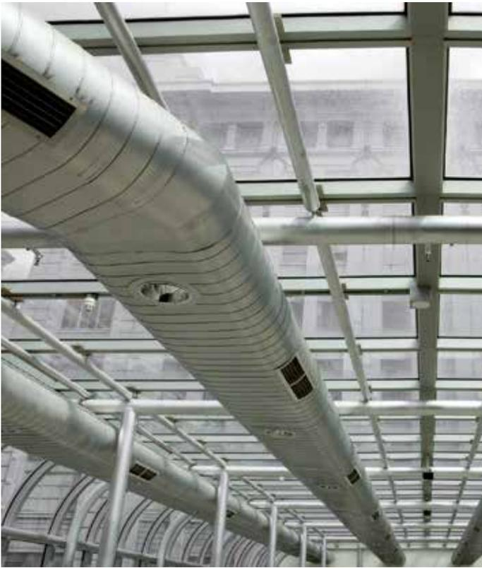
These systems are designed to maintain environment temperature and humidity at desired levels by varying flow rate in accordance with parameters such as the presence of people and internal and external temperature differences.
